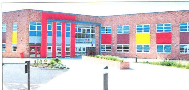
OFFICIALLY OPEN: Speeches and tours marked the official opening of the new £8million facilities at Ormiston Venture Academy in Gorleston.
